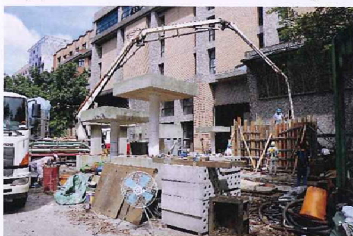
(c) 混凝土梁柱灌漿(105/10/17)
