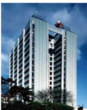
Figure 1 Before the retrofit
