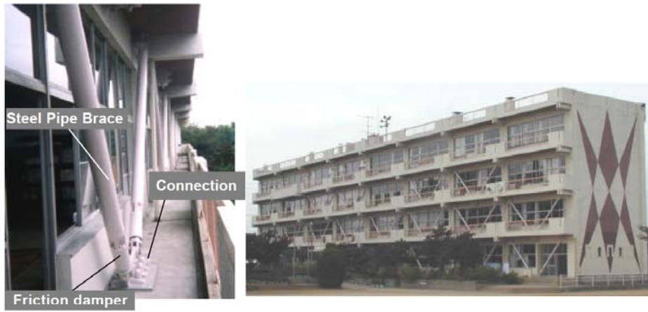
Photo. 4 Application to a balconied school building
