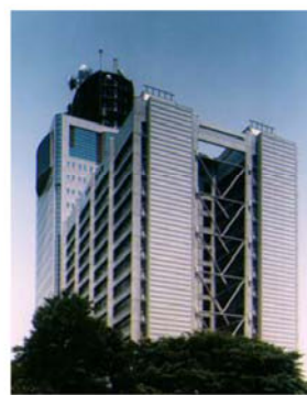
Figure 2 After the retrofit
