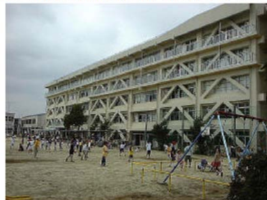
d) Elementary School Building (with Balconies)
