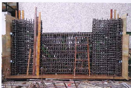
(a) 鋼筋組立(105/10/06~105/10/13)
